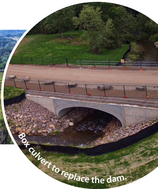
Before (left) and after (right) decommissioning of the Albion Hills Pond.
