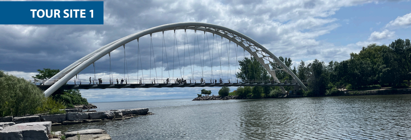
View of Humber Bay Arch Bridge at the mouth of the Humber River.
