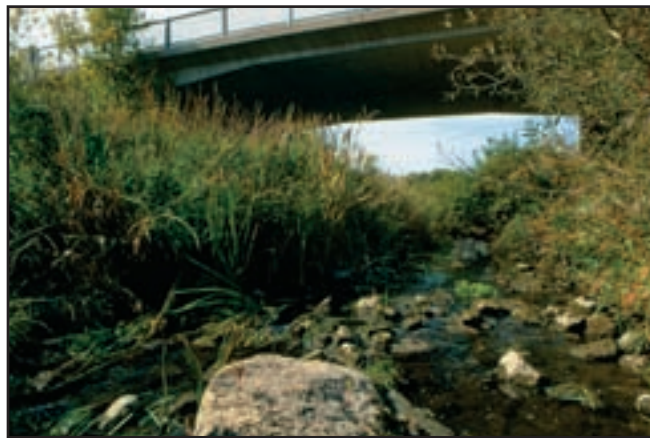
Natural watercourse under bridge.
