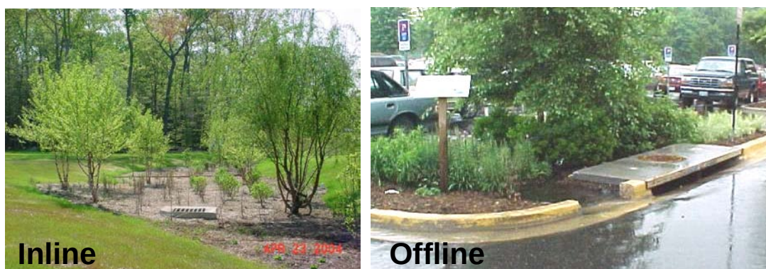
Figure 4.5.9 Examples of inline and offline bioretention
