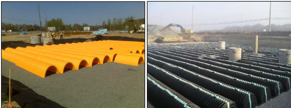
Figure 4.4.2 Infiltration chambers under construction in commercial developments
