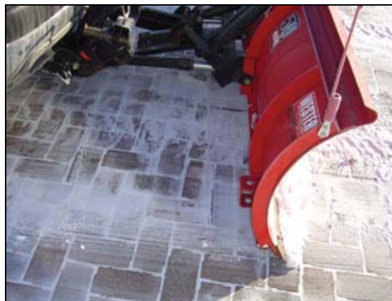
Figure 4.7.8 Permeable pavement is plowed like any other pavement.
