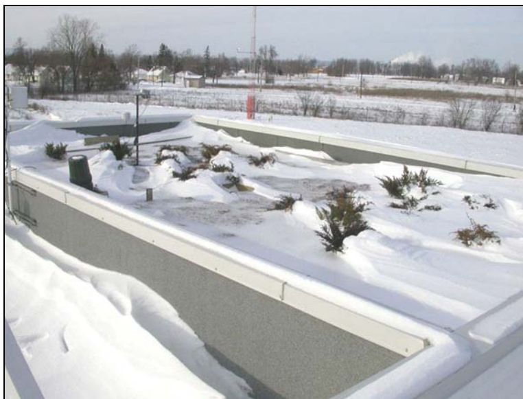
Figure 4.2.2 A green roof during winter
