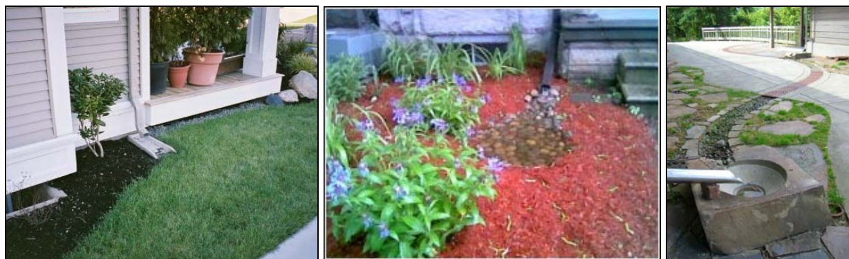
Figure 4.3.1 Examples of disconnected downspouts draining to a splash pad (left), a rain garden (centre) and an infiltration trench (right)
