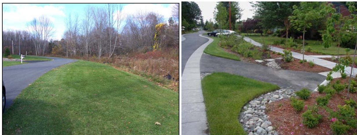
Figure 4.6.1 Filter strips along a residential road and as pretreatment to a dry swale
