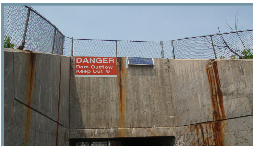
Stouffville Dam Spillway
