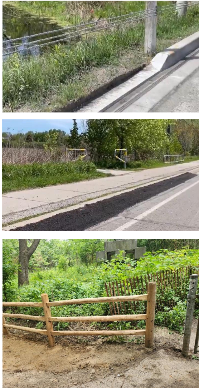
Figure 4. From top to bottom: a curb cut implemented in Richmond Hill; a curb ramp constructed with asphalt also in Richmond Hill; and an example of post and paddle fencing.
