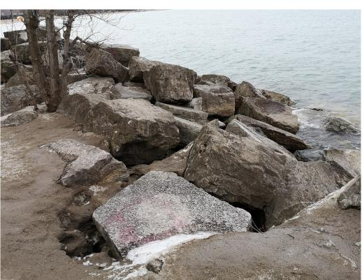
Waves have moved stones out of place, reducing shoreline stability and causing erosion of the park.
