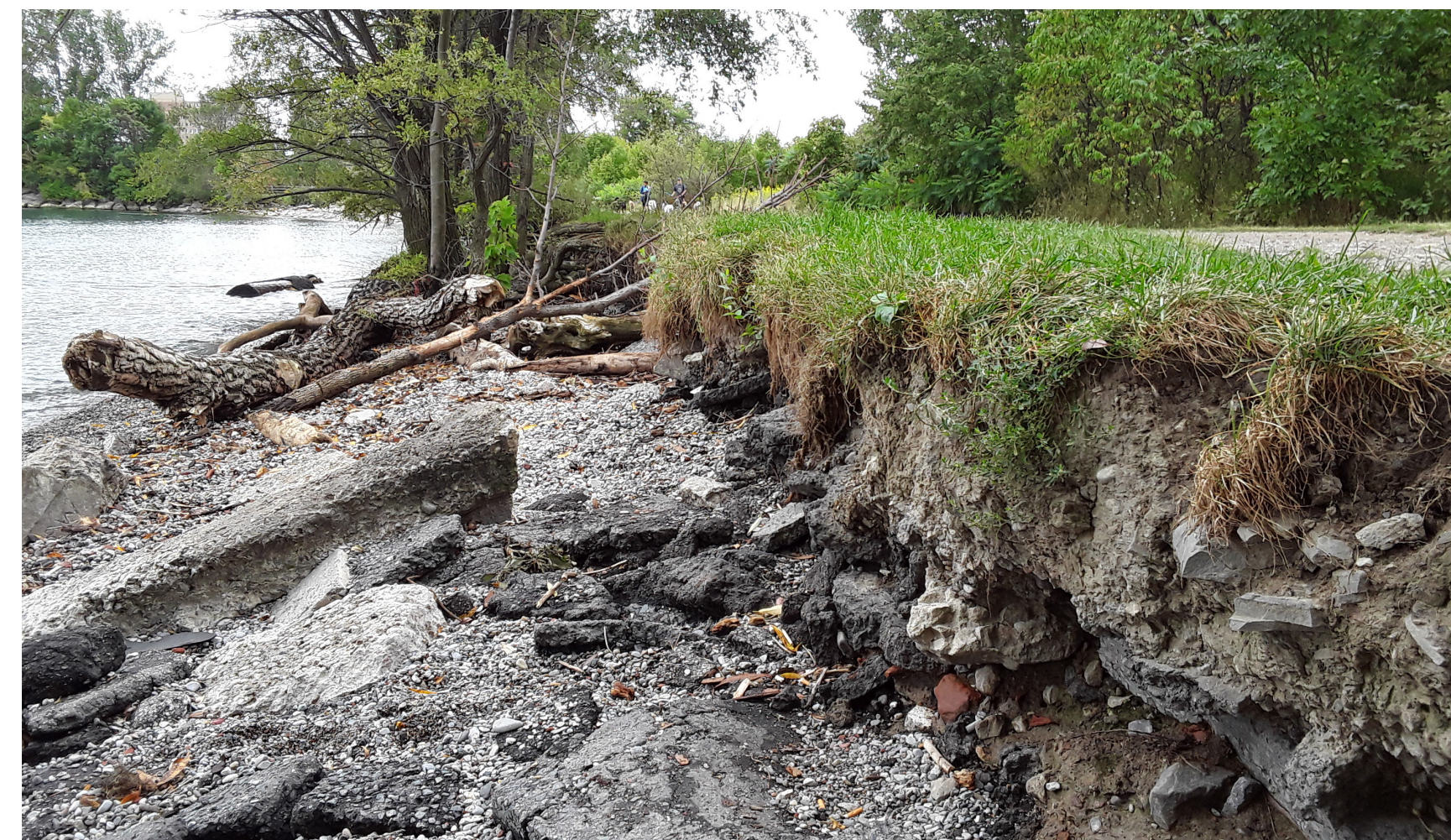
Waves have eroded banks placing trails and park infrastructure at risk. These areas need to be repaired to protect parkland and trails.
