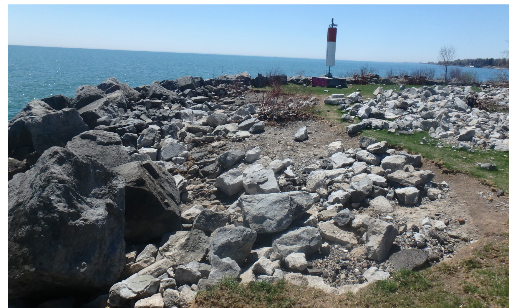
Waves have shifted rocks so they no longer provide proper protection, and parkland is starting to erode.
