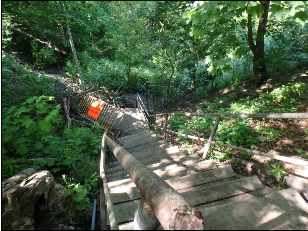
Figure 5: Displacement of soil across the lower landing and leaning guard rails of the municipally owned staircase (TRCA, 2017).
