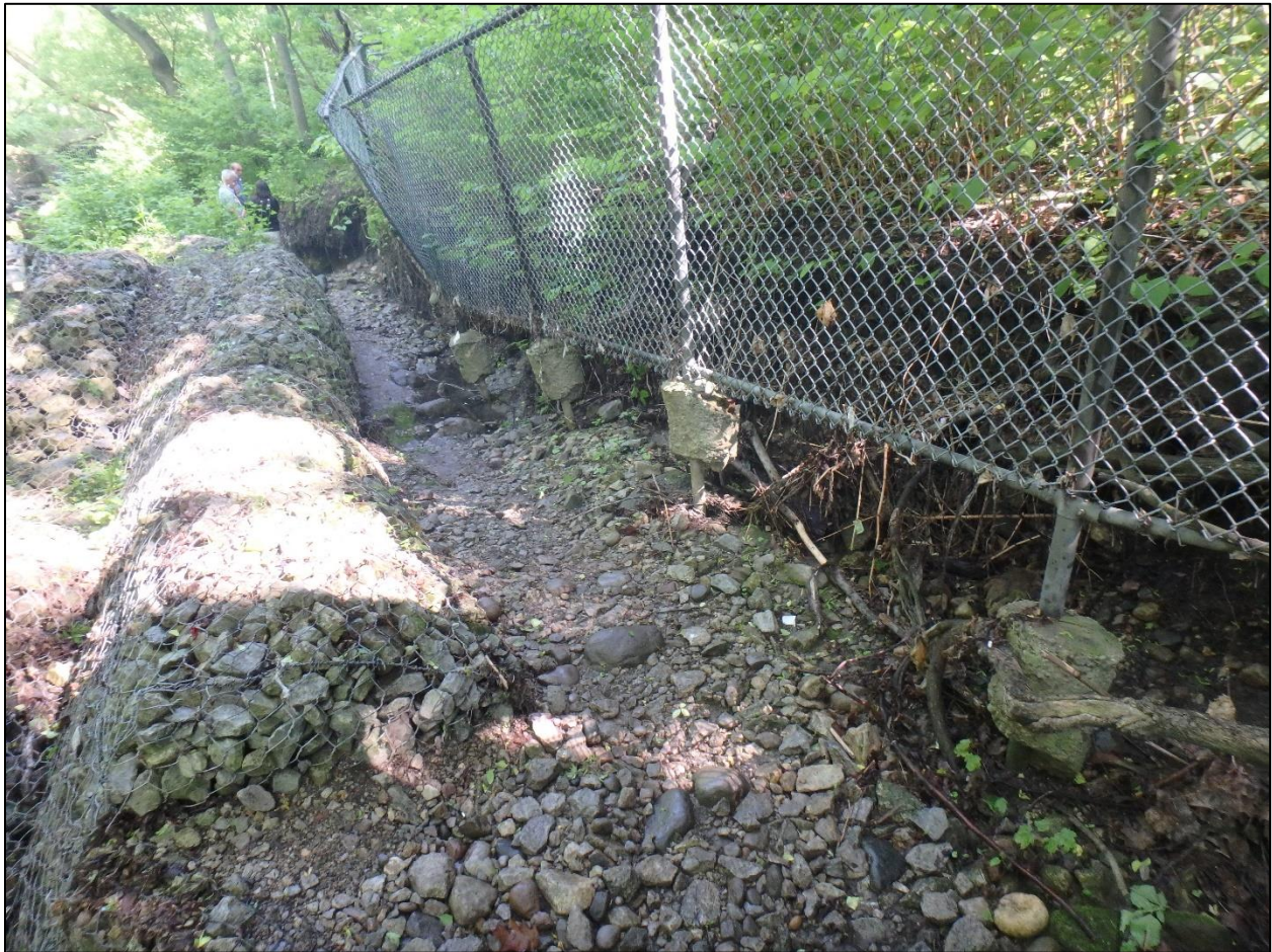
Figure 10: Elevated flows within Yellow Creek have outflanked the existing gabion stone bank structure, impacting a property fence line and eroding the toe of slope behind (TRCA, 2017).
