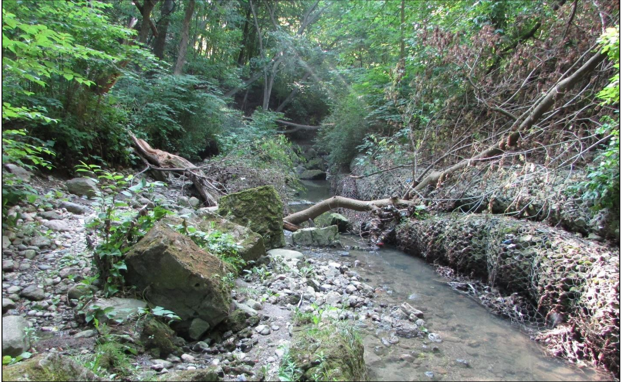
Figure 8: Looking downstream (south) along Yellow Creek, bank stabilization structures have been degraded and displaced by the forces of erosion (TRCA, 2019).
