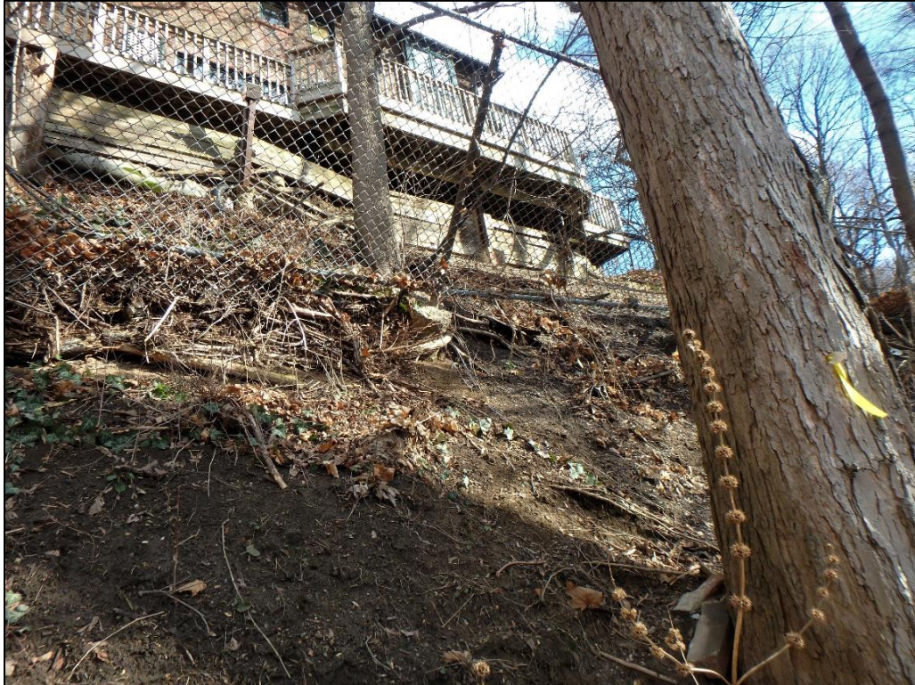
Figure 6: A failing retaining wall below a private residential dwelling can be seen above; the bare upper slope below this property is also indicative of active slope erosion (TRCA, 2016).
