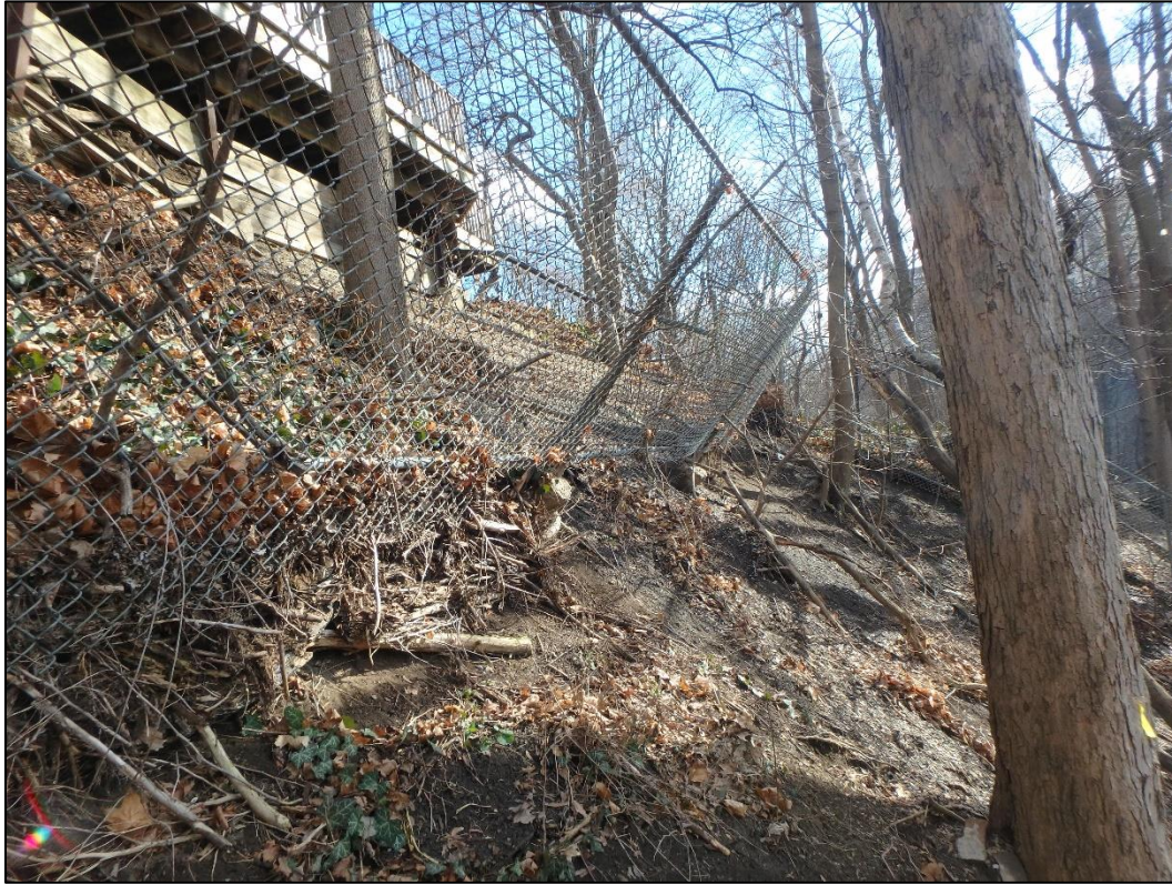
Figure 7: Slope instability and active erosion along the east valley wall have caused a property fence to lean and exposed its footings (TRCA, 2016).
