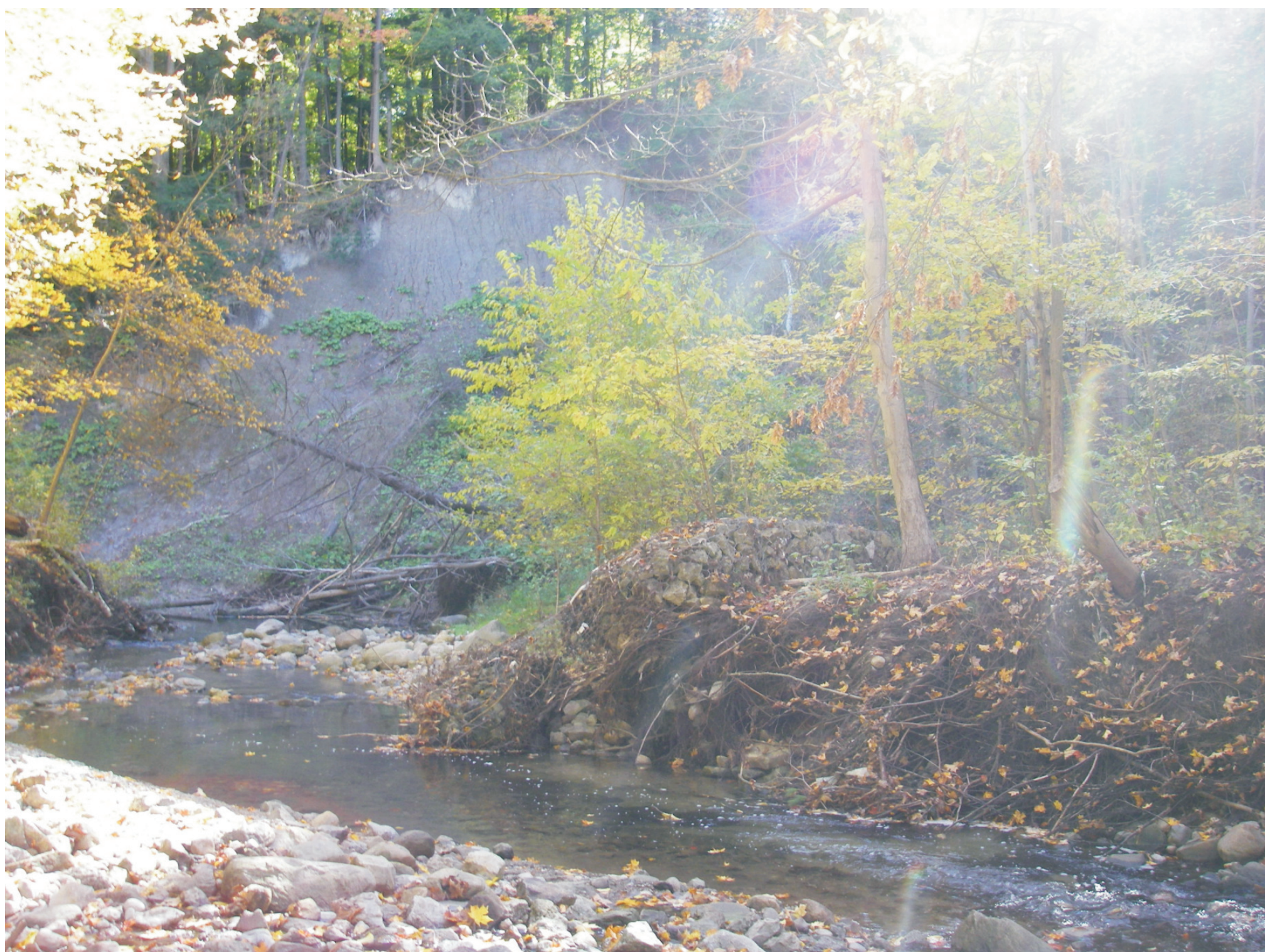
Failed gabion baskets and valley slope erosion.
