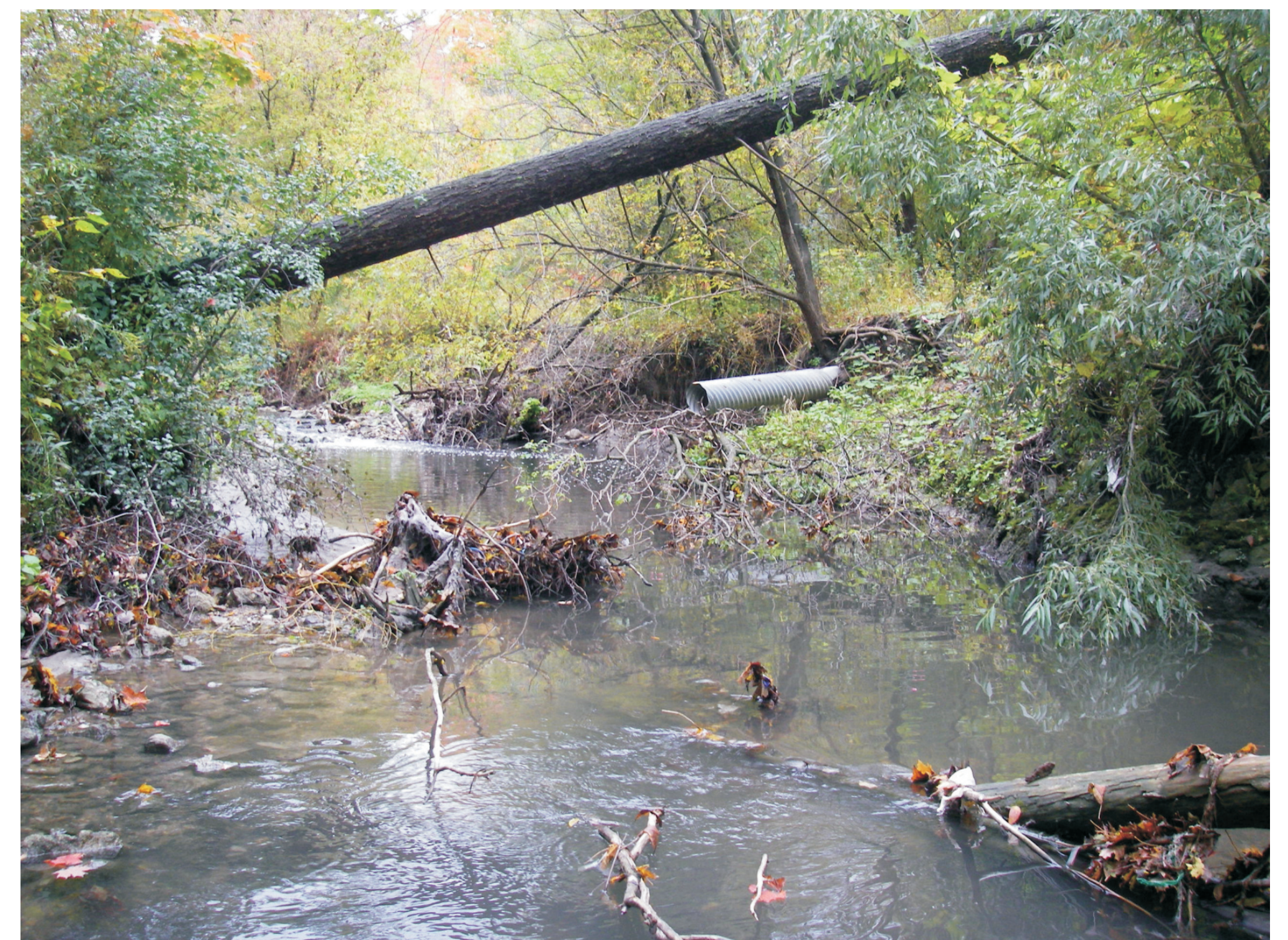
Widening channel and exposed infrastructure.
