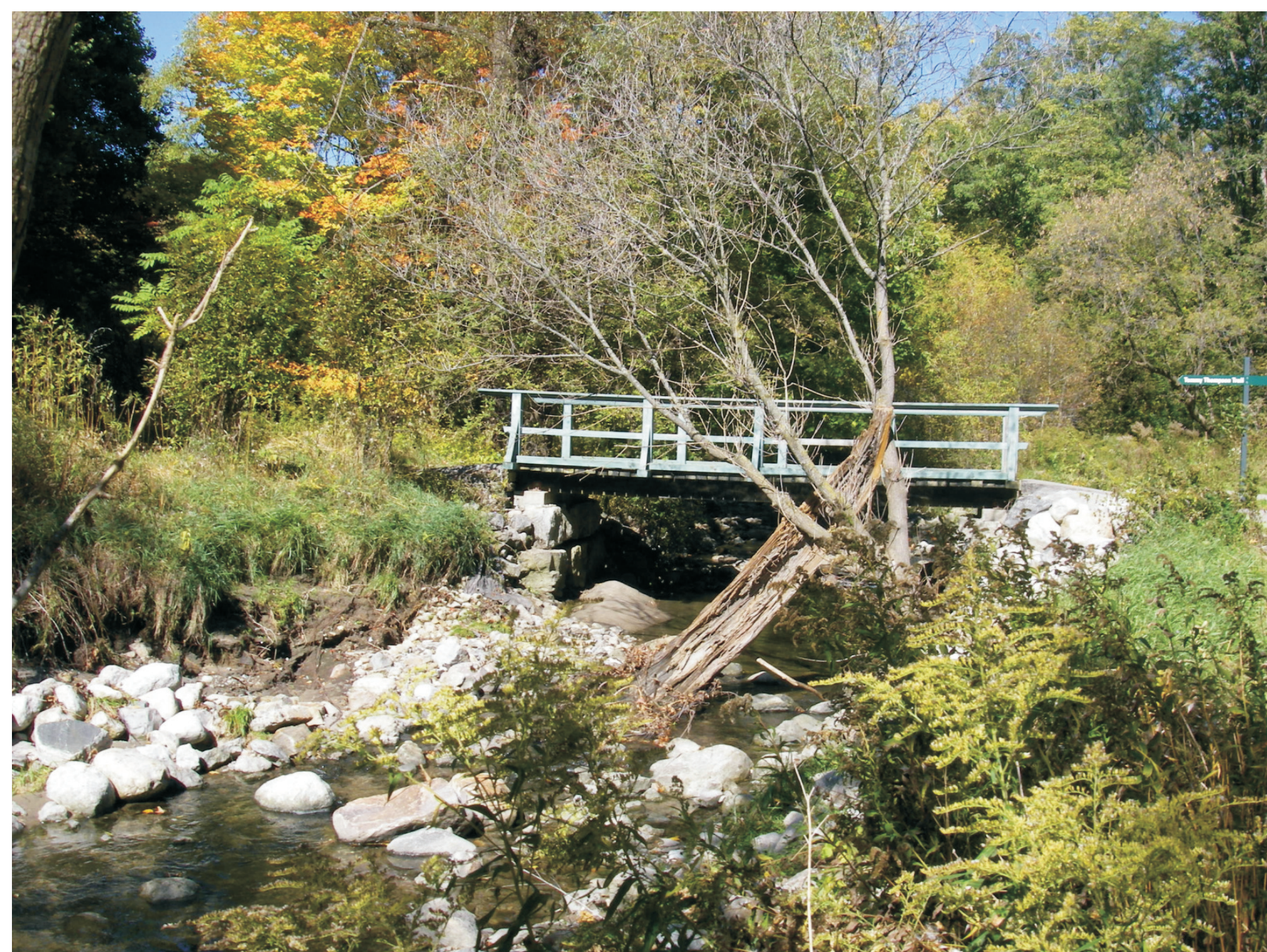
Erosion threatening a pedestrian bridge.
