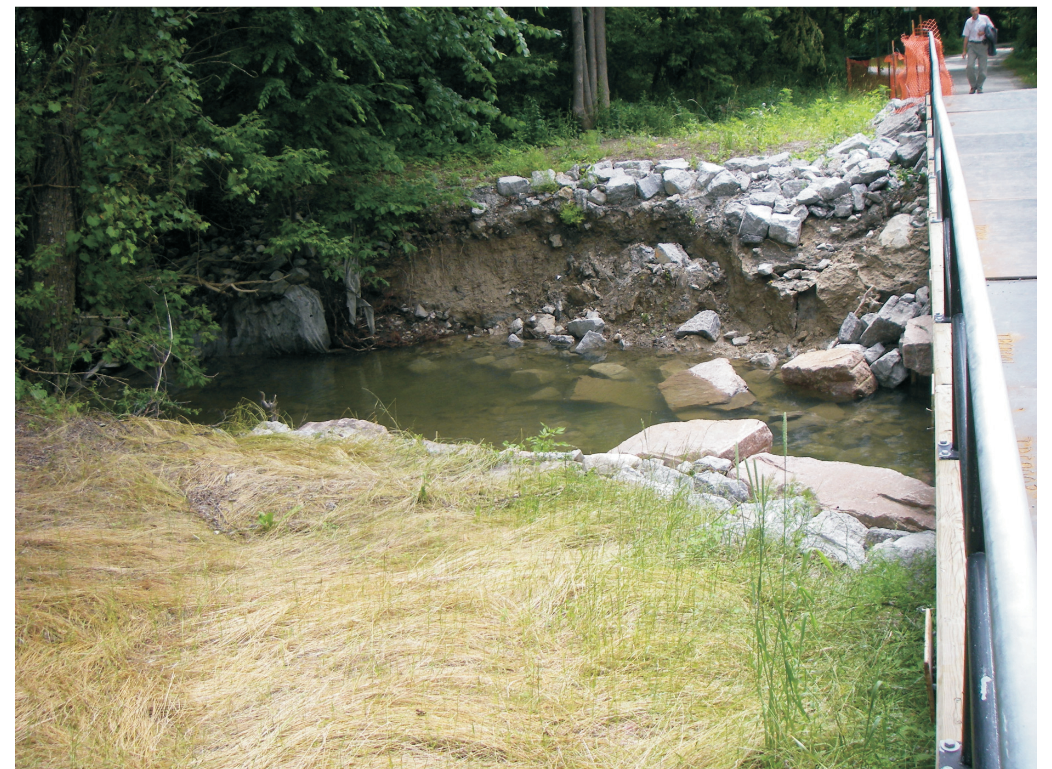
Erosion at temporary bridge repairs.
