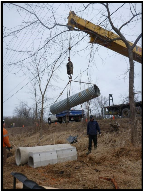
Figure 7 – Crane positioning culverts
