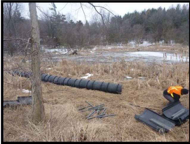
Figure 3 –Staff installing ACO directional fence
