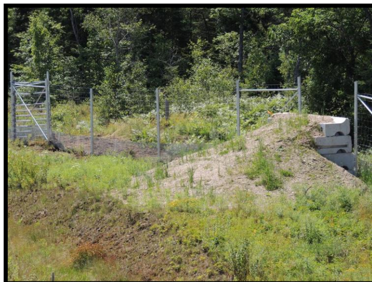
Figure 68. Directional fencing, chain link with hardware cloth, one-way entry from road.
