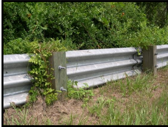
Figure 64. Directional wildlife fence, buried guardrail (Photo Credit: Aresco MJ).
