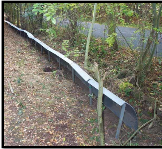
Figure 66. Directional wildlife fence, ACO one-way wildlife fence.
