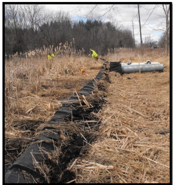
Figure 6 – ACO fence with banked natural material
