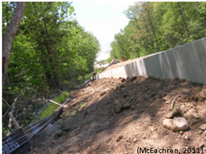
Image 6: Permanent Concrete Wall Directing Wildlife to Underpass
