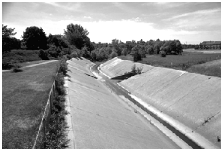
Concrete lined section of Etobicoke Creek
