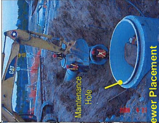
Storm Sewer Connections
