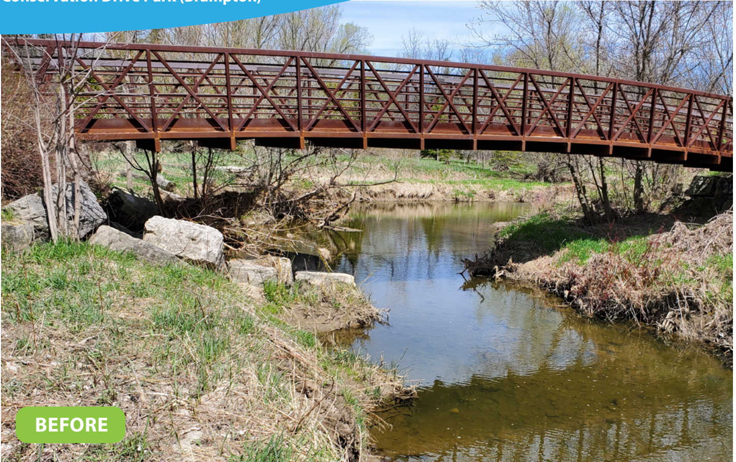
FIGURE 18: Before and After, Stream Restoration at Conservation Drive Park (Brampton)
