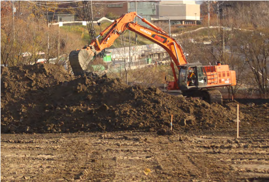
Conventional topsoil stripping and stockpiling practices tend to compact the soil and deplete it of beneficial soil organisms which results in stockpiles that are either poor or highly variable in quality. Source: Dean Young
