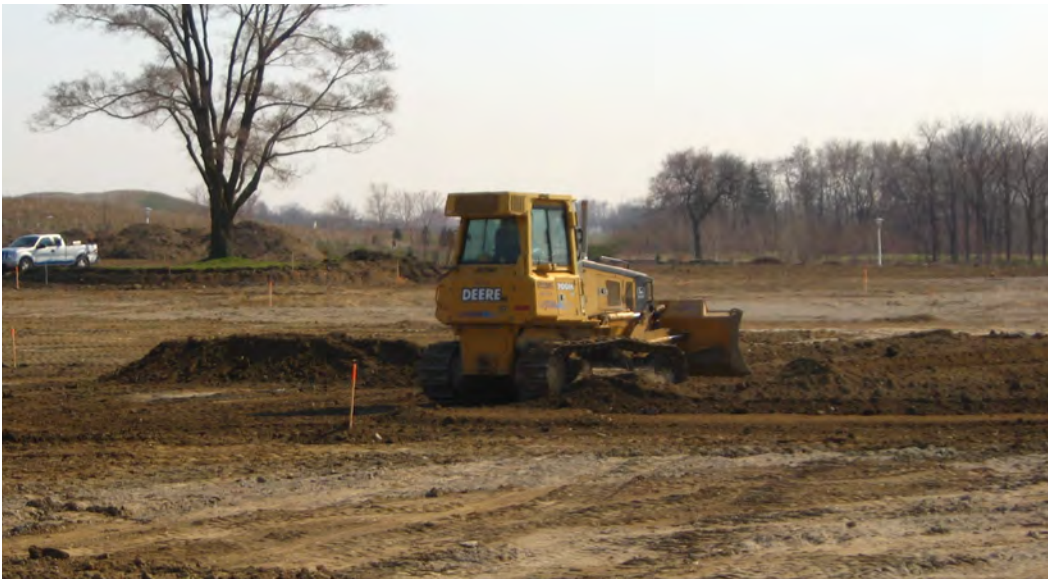
Topsoil being reapplied to a construction site with a tracked low ground pressure (LGP) bulldozer. Source: D. Young
