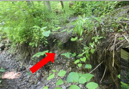
Scouring along channel of Yellow Creek at toe of Slope
