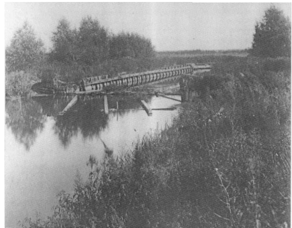
Figure 7: The Toronto Dry Dock looking south from the old Don River near Cherry Street in 1898. The structure appears to have been built of timber cribs.
