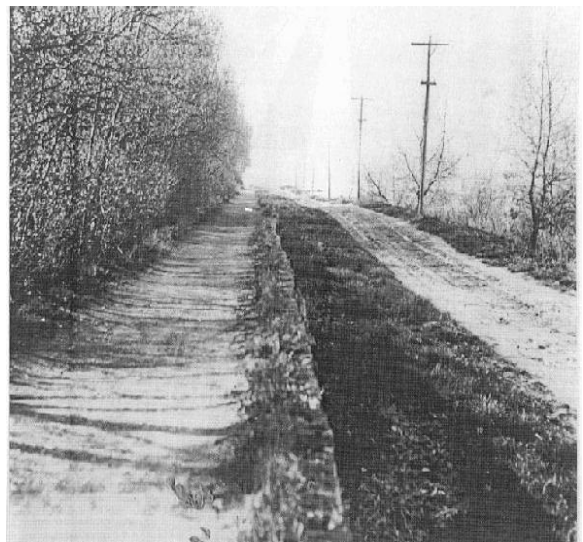
Figure 8: The Government Breakwater in 1909. The double rows of sheet piling are indicated by the line of trees on the left and the line between the light and dark ground in the middle.
