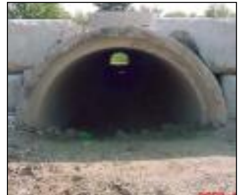
Figure 13. Concrete elliptical ecopassage (photo credit: Ecoplans Limited).
