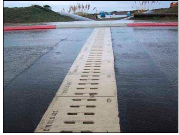
Figure 11. ACO Wildlife tunnel flush with road surface.
