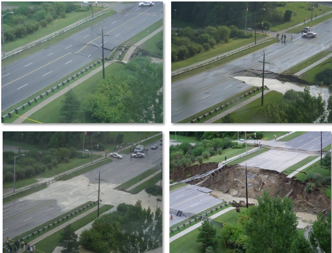
Figure 43: Finch Avenue culvert failure August 19 th , 2005 Toronto, >125mm in less than 1 hour.
