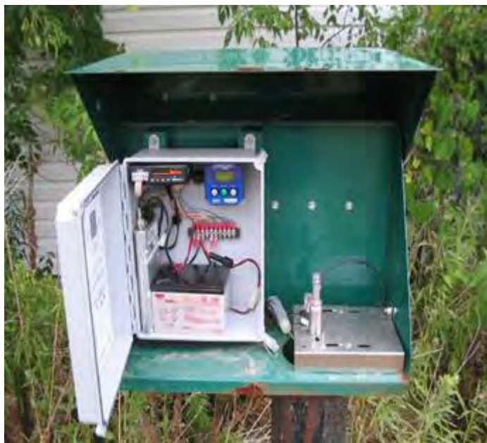
Figure 34. PGMN well with telemetry equipment and dedicated pump installed
